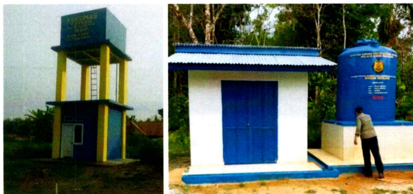
Gambar I.2 Gambar Sumur Pompa
