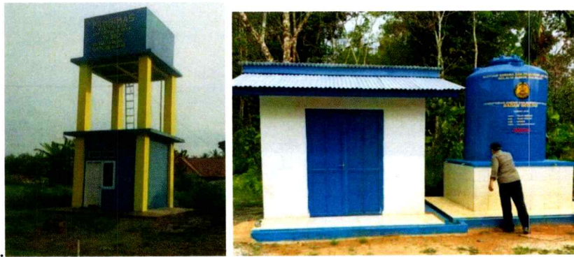
Gambar II.2 Contoh Sumur Pompa
